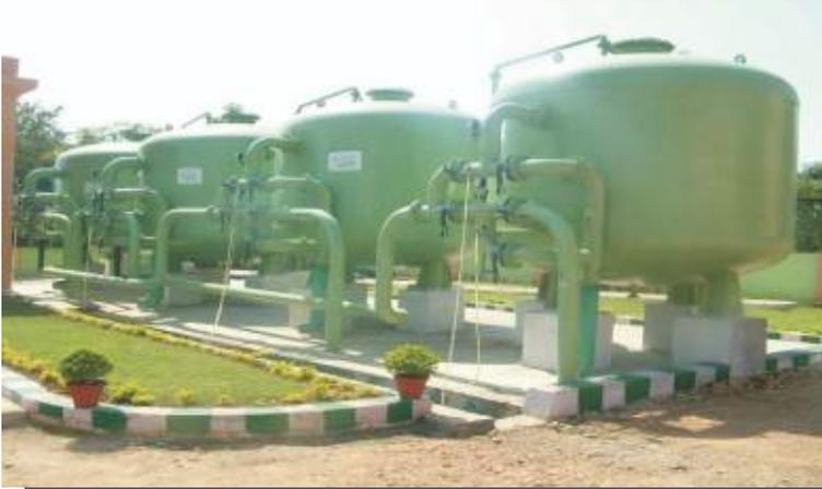
**Pressure Filter** is a closed cylindrical vessel either vertical or horizontal (mostly vertical) containing the filter media over a collector system. Water flows from top downwards percolating through the media and is drawn off through the collector system at the bottom. Cycle of operation include back washing with or without air scouring, short rinse to waste and return to operation.
